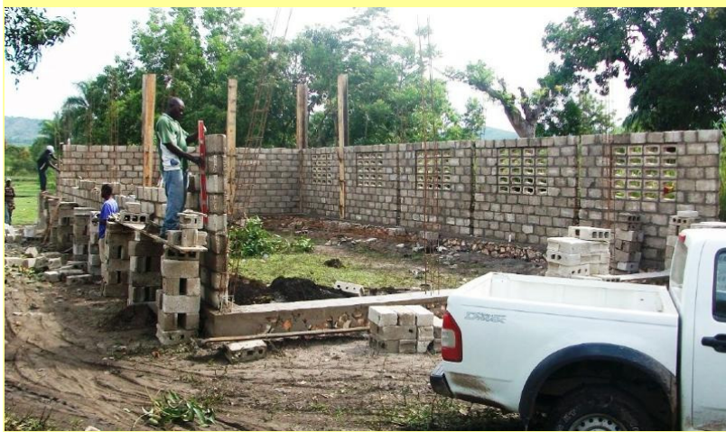
Progress on the church as of June 9th
